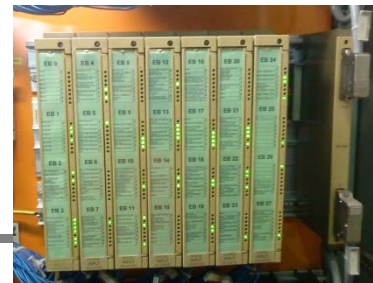
Expansion racks with digital input/output cards
