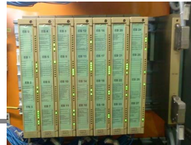
Expansion racks with digital input/output cards
